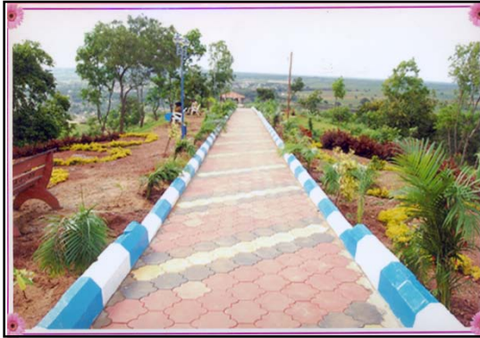
Paves and Kerb Stones for Pathway,
