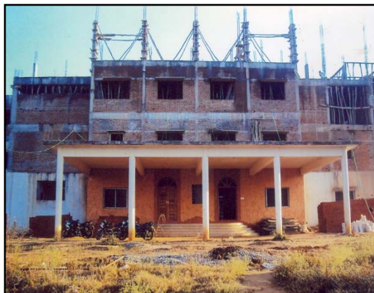
Construction of Jain Yatri Nivas
