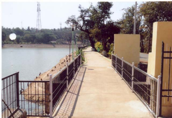
Tank Development including desilting, stone pitching and Island creation.
