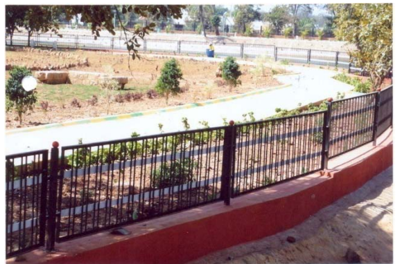
Foot path & railings
