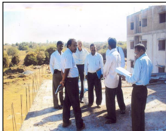
Construction of Jain Yatri Nivas
