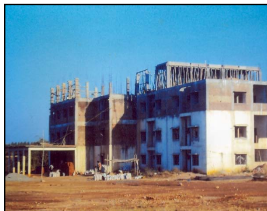
Construction of Jain Yatri Nivas
